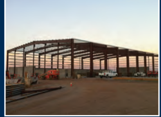
Metal Building Erection in Process
